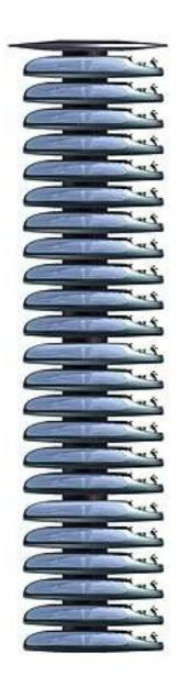
This tower has a height of 250 meters and 59 floors mounted in a concrete core which will serve as a rotating shaft. The floors will be preassembled and then attached to the core of the building.
